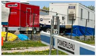
Photos of a construction washroom trailer taken at the Pomerleau construction site at Majors Hill Park in Ottawa, Ontario May 2023. Standard units include flushing toilets with a porcelain tank, a counter, a sink, a porcelain urinal, a mirror, a window, an exterior lock, a light, air conditioning, air exchanger and heating.
