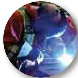
Welders weld ferrous and nonferrous metals on plates and pipes, using SMAW, GTAW, and FCAW processes and manual or semi-automatic welding equipment. They use flame-cutting, brazing, and air-arcing equipment. Welders must be able to read simple instructions and follow them precisely. Welders have great manual dexterity and must be agile and in good physical health. They also have analytical ability and an understanding of computerized machinery.
